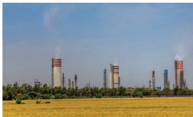
Figure 1. Photograph of CFCL plant
