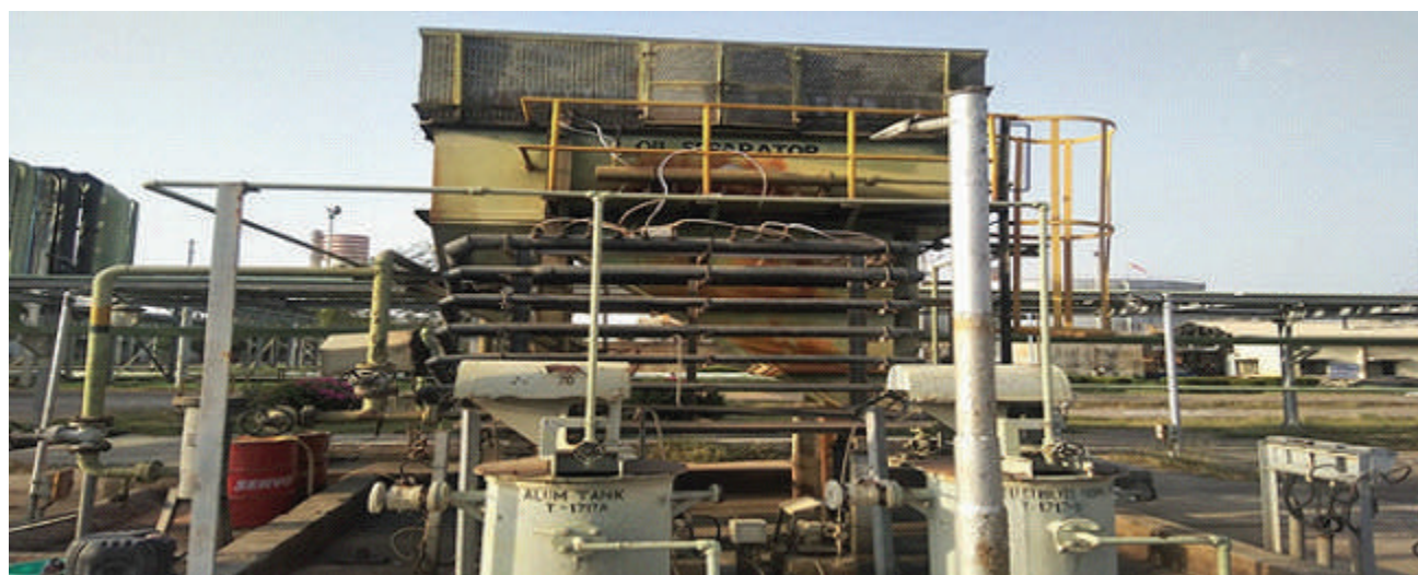
Figure 4. Treatment of oily waste water
