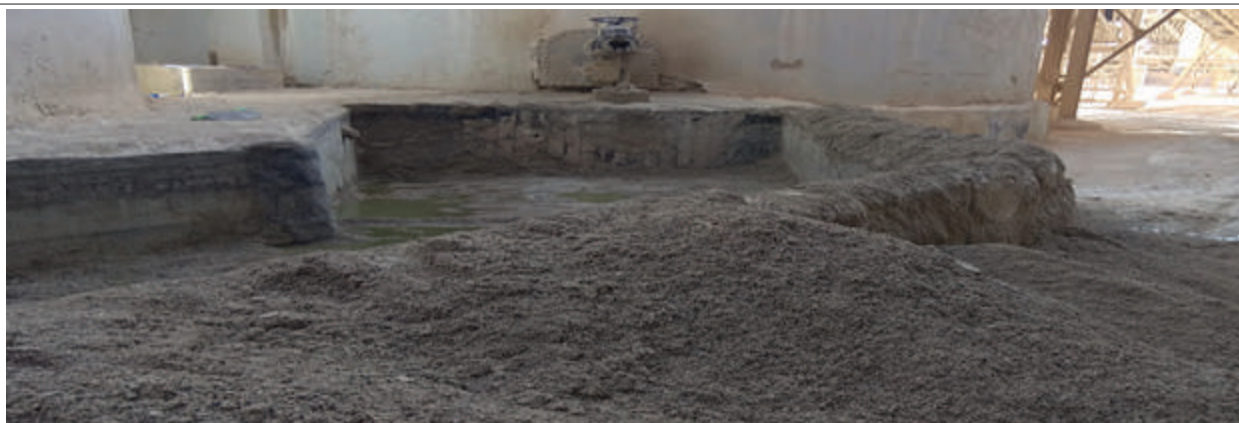
Figure 2. Reactor draining facility to remove settled heavier particles from vessels bottom
