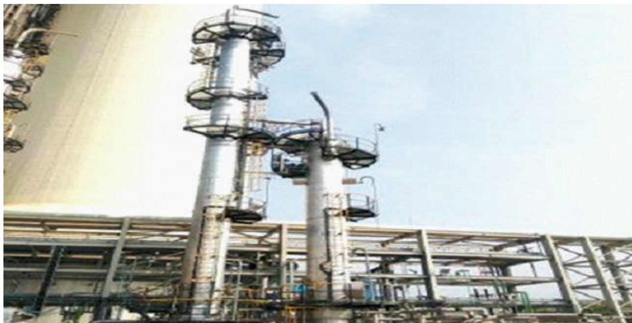
Figure 3. Deep hydrolyzer in urea plant
